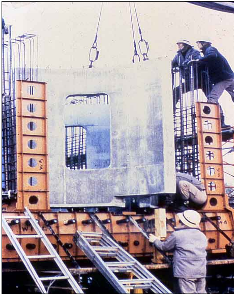
Testing of precast honeycomb elements for LNG platform construction.
