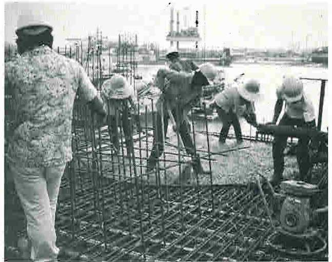
Top left: Workers shown forming barge cylinders. Bottom left: Precast circular and star-shaped slabs help form top deck. Top right: Here construction crew pours top deck. Bottom right: Stressing operations at stern of barge.
