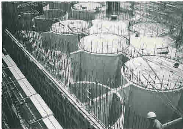
Top left: Workers shown forming barge cylinders. Bottom left: Precast circular and star-shaped slabs help form top deck. Top right: Here construction crew pours top deck. Bottom right: Stressing operations at stern of barge.
