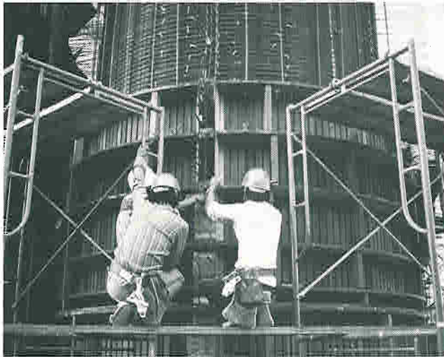
Top left: Workers shown forming barge cylinders. Bottom left: Precast circular and star-shaped slabs help form top deck. Top right: Here construction crew pours top deck. Bottom right: Stressing operations at stern of barge.
